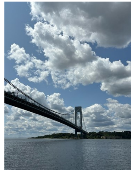
Verrazano Narrows Bridge, photo by Doug Henry
