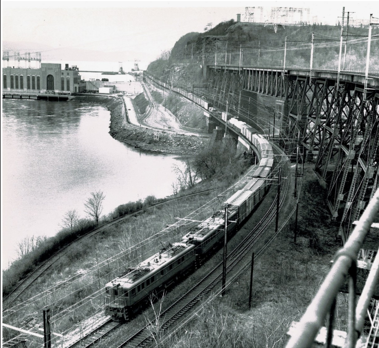
Left: The iconic Safe Harbor Dam in 1962.
