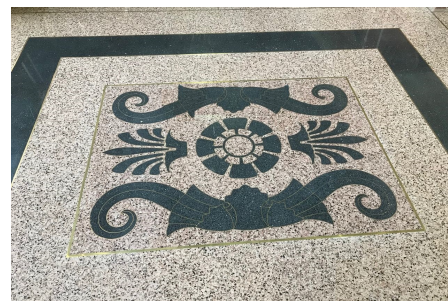
THE ORIGINAL 1935 ERA FLOORS IN NEWARK PENN STATION ARE AMONG THE FEATURES INCLUDED IN A $160 MILLION RENOVATION AND REHABILITATION.
