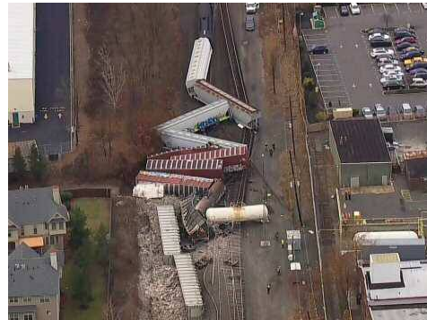
AFTERMATH OF CSX DERAILMENT IN UNION, NEW JERSEY NBC4NEW YORK
