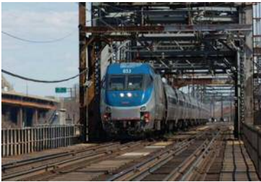
THE EXISTING PORTAL BRIDGE WAS BUILT IN 1910 - AMTRAK PHOTO.
