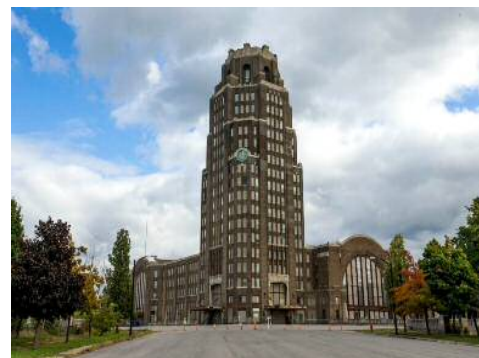
BUFFALO'S CENTRAL TERMINAL IS A POTENTIAL SITE FOR THE NEW AMTRAK STATION - PHOTO BY DEREK GEE, THE BUFFALO NEWS.
