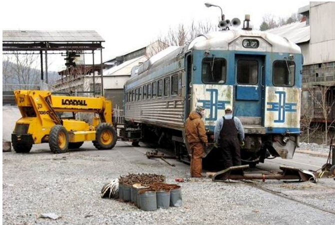
WORKERS PREPARE RDC No. 9167 FOR RESTORATION BELLEFONTE HISTORICAL RAILROAD SOCIETY
