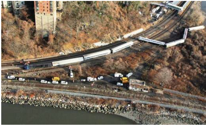
OVERHEAD VIEW OF THE DERAILMENT SITE ON DEC. 1, 2013. SPUYTEN DUUVIL STATION IS AT THE TOP RIGHT. AMTRAK'S WEST SIDE LINE IS AT THE BOTTOM. NTSB PHOTO.
